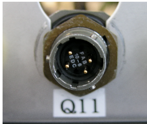
Figure 6: Connector with Missing Pins (Ericsson Cable)
