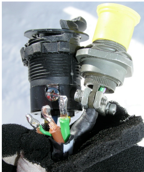
Figure 1: Broken and Missing Marincos Connectors on JDR Cable
