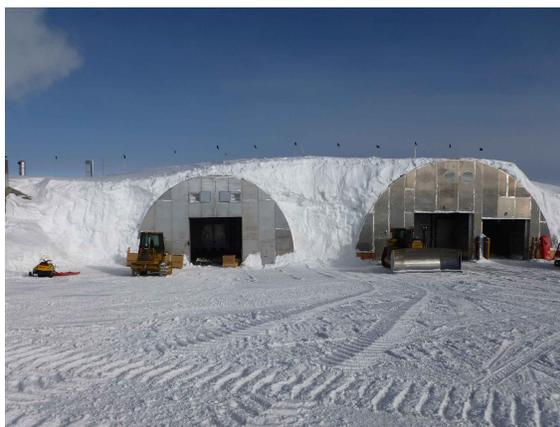
(a) Cargo (left) and garage (right) arches; the arches reach peak heights of 8.3 (left) and 9.8 m
